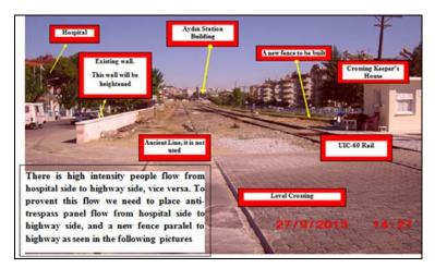
Figure 5.5-6 Measure 7: Installation of anti-trespass panels in the second point.
