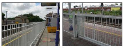
Figure 5.6-1: Mid-platform fencing that has been installed at one of our trial stations (left). A sliding gate in the fencing to allow access to the platform when necessary (right).
