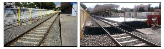
Figure 5.5-7 Measure 7: Before/after Anti-trespass panels.
